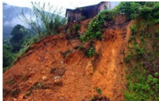
Hillside after rainfall
