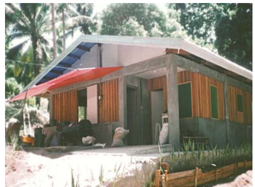
Figure 13. The newly established arrowroot processing plant.
